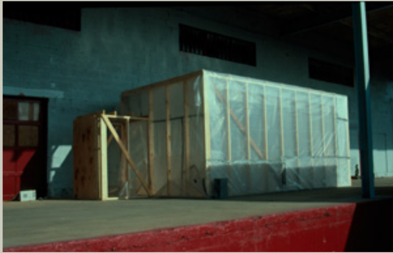
Asbestos decontamination chamber
