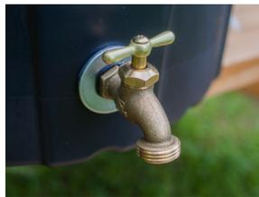
**Step 5:** Add an O-ring and washer to your spigot inlet and screw it in. Add a bead of caulk behind the washer and allow to dry to make it watertight.
