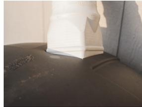
**Step 3:** Plug the gutter spout into your rain barrel lid to begin collecting water.
