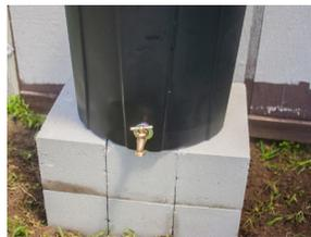
**Step 6:** Your rain barrel is now ready to go! Rain will run off your roof into the barrel and be ready whenever you need to fill your watering can. You can even hook up your hose to the spigot if you want to!
